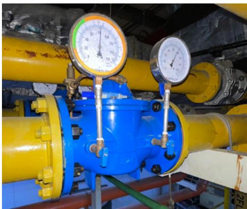
The Company has implemented the installation of a pressure regulator to separate the compressed air system into two levels : High Pressure and Low Pressure. This optimization ensures appropriate usage and prevents unnecessary energy consumption. As a result, one air compressor (500 Hp, 373 kW) has been decommissioned, leading to a reduction in electricity consumption by 174 MWh, cost savings of THB 0.8 million, and a reduction in GHG emissions by 480 tonCO<sub>2</sub> e.
